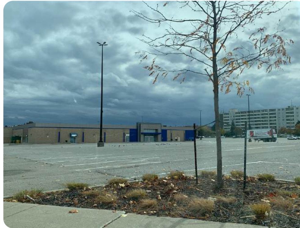
On Kenora Avenue looking southeast towards the west side of the existing Eastgate Square
